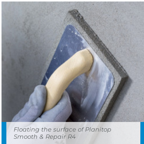
Applying Planitop Smooth & Repair R4 with a trowel
