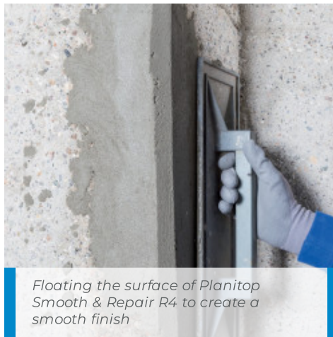
Applying Planitop Smooth & Repair R4 with a trowel
