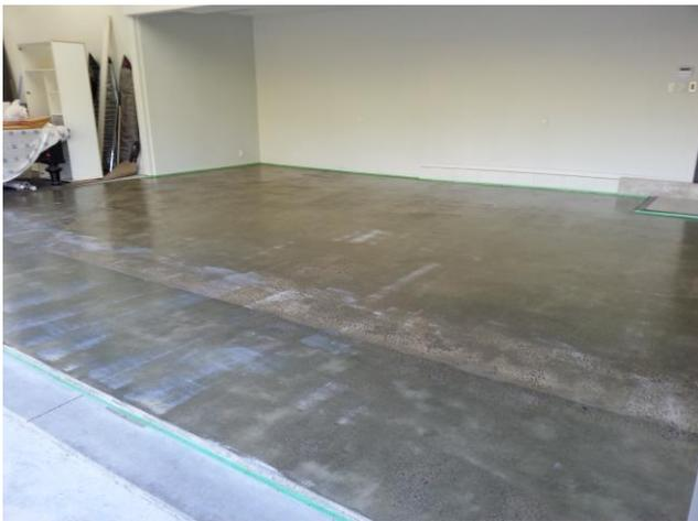
**DESCRIPTION:** A water based speciality acrylic co-polymer sealer, incorporating nanotechnology that aids binding and penetrating friable substrates. High penetration and wet out prepares concrete surfaces to more effectively key high solids low penetrating top coats.
